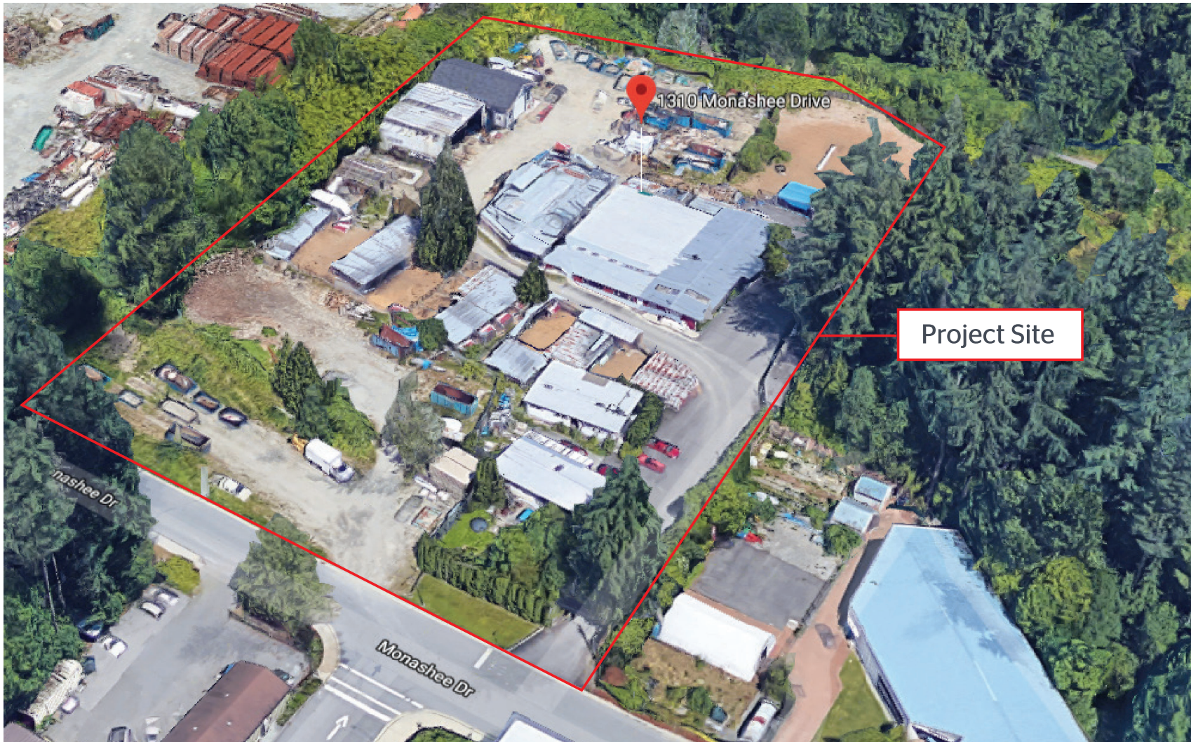
Aerial - South West
